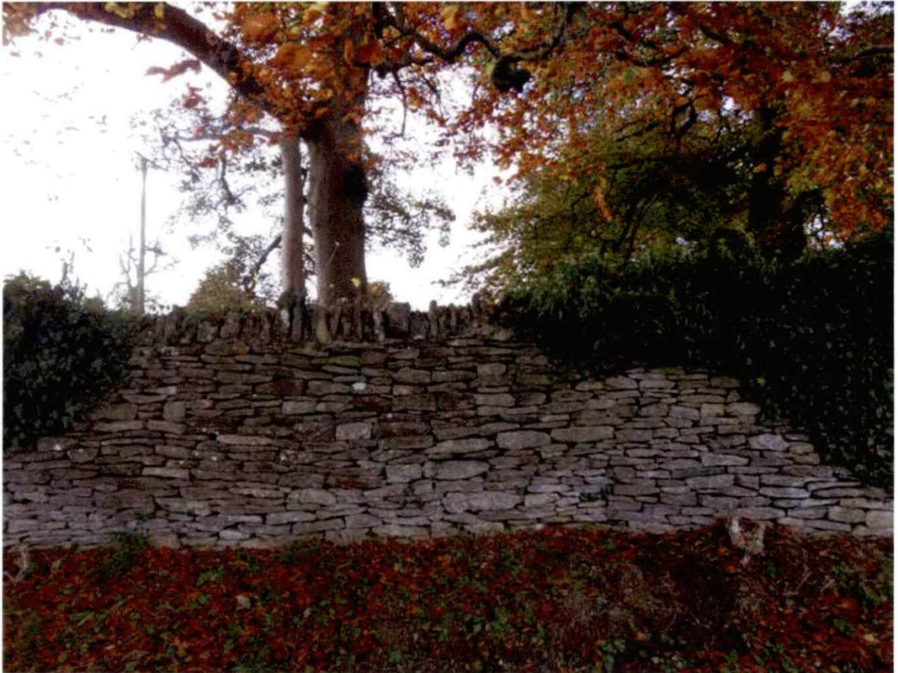
7. View from footpath on Maugersbury Road.
